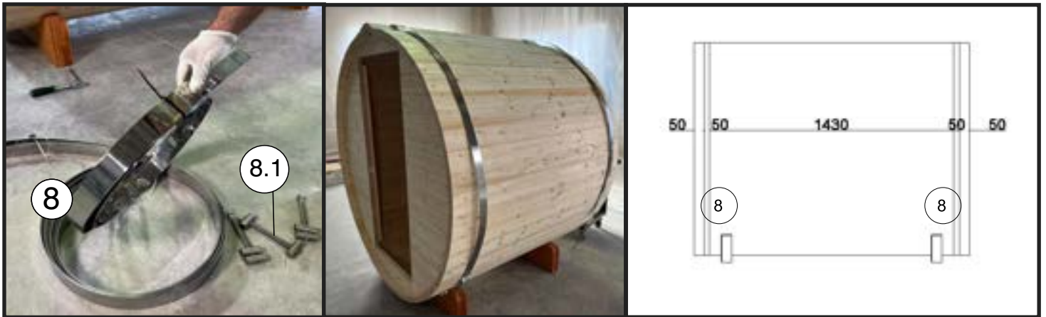
7.3 Tighten the bands with the help of a hex key.
